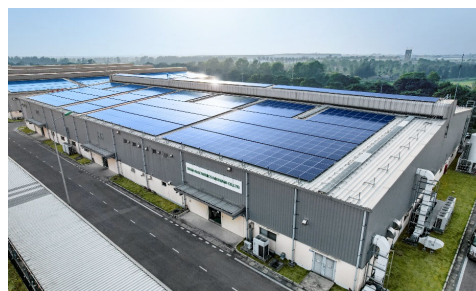
Solar panels installed at Vietnam factory
