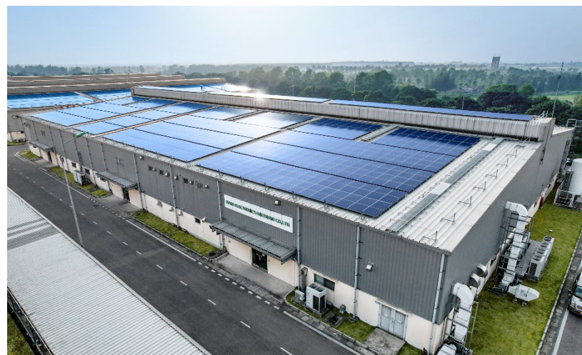
Solar panels installed at Vietnam factory
